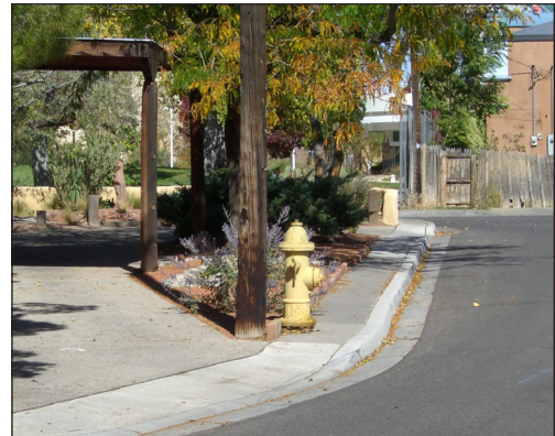
Fire hydrant obstructing very narrow sidewalk
