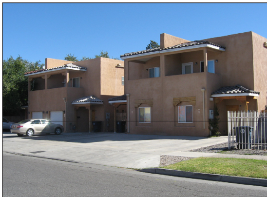
Townhomes along 11th Street with no area left for landscaping in the front setback
