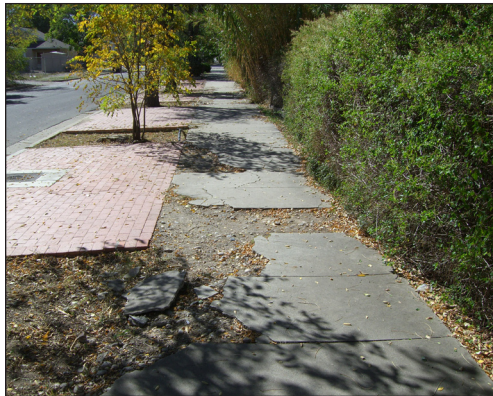
Deteriorated sidewalk
